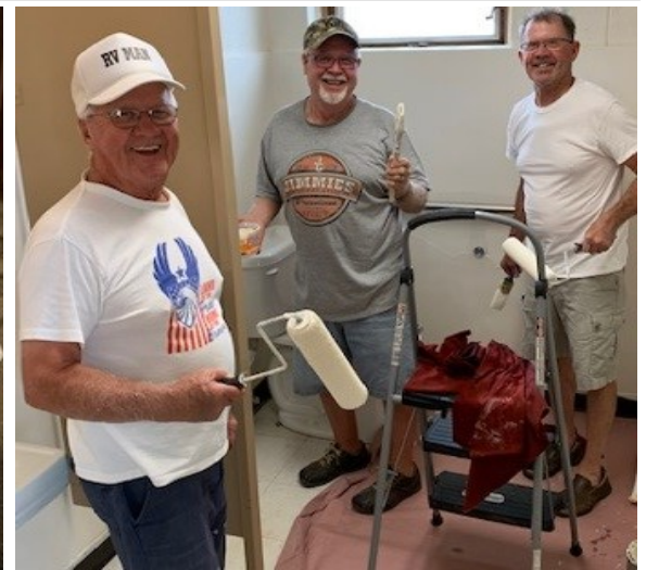
Refreshing the Restrooms off of the lounge
