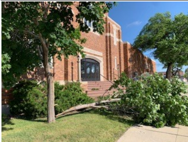
Storm Damage from June 7th Winds
